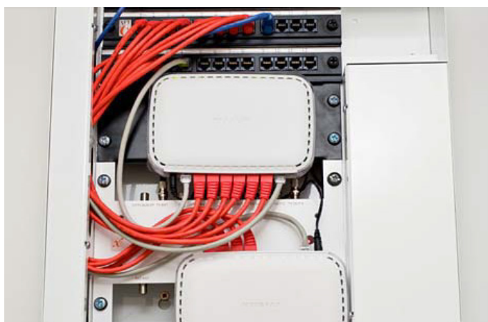
Connectix Home cabinet, TV distribution unit and Home patch panels
